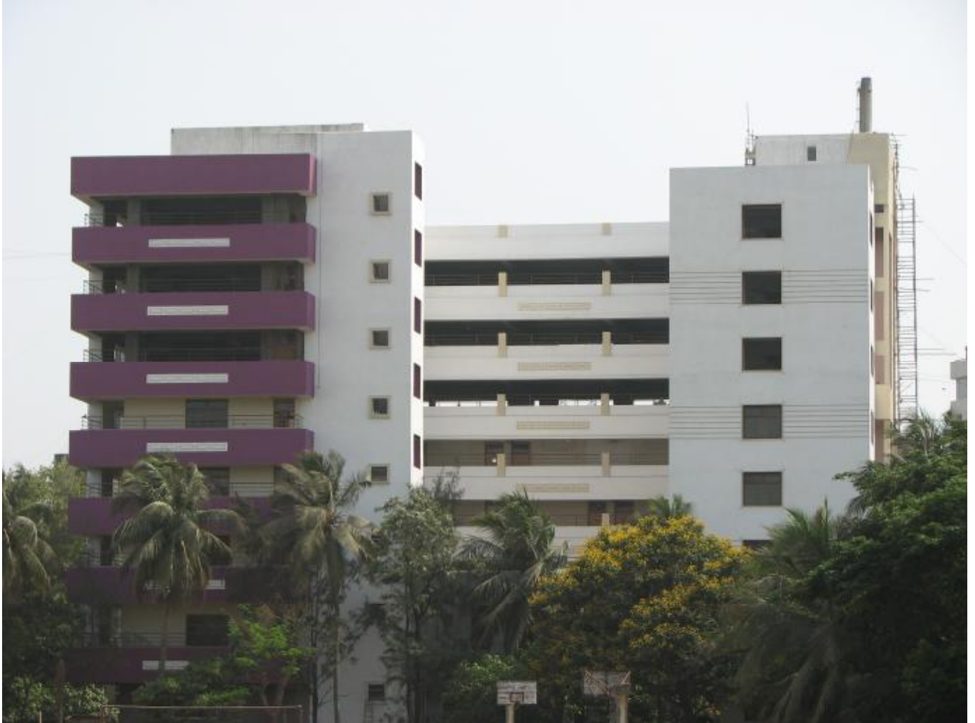
New Building under construction in Ruparel Campus
